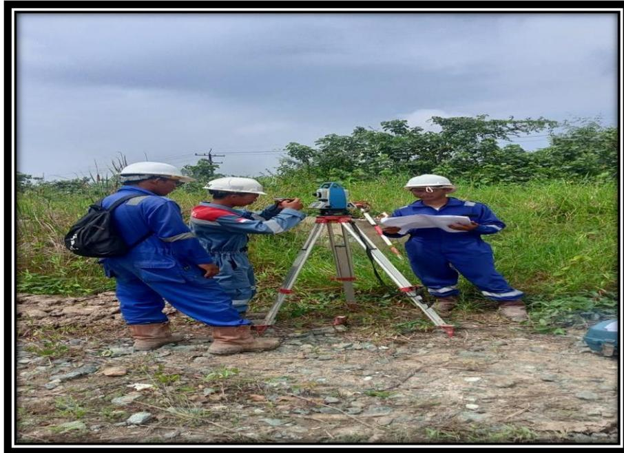
Gambar 7. Pengukuran *Staking Out*
